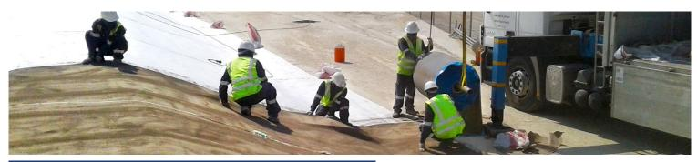
CC Hydro<sup>™</sup> Geosynthetic Cementitious Composite Barrier (GCCB) is a revolutionary new containment product from Concrete Canvas Ltd.
