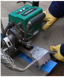
CC Hydro™ can be rapidly unrolled to provide a high impermeability channel, flume or canal lining for drainage, irrigation or hydroelectric schemes; providing flow characteristics similar to smooth concrete (manning's = 0.011) is 5 times as abrasion resistant as standard OPC concrete - please refer to CCH Data Sheet.
