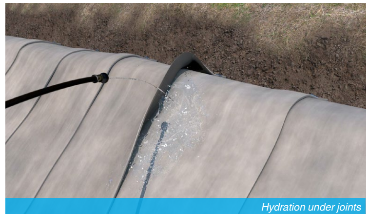
Overlap in direction of water flow
