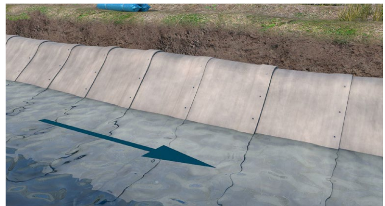
Overlap in direction of water flow
