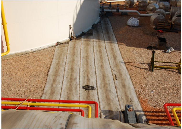
CC was unrolled down the slope and along the tank farm floor
