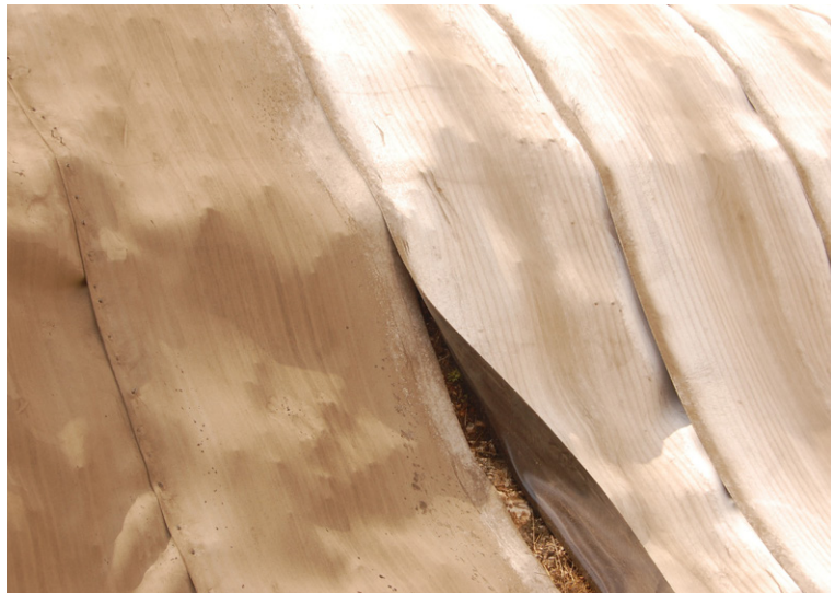
Additional layers were overlapped by 100mm
