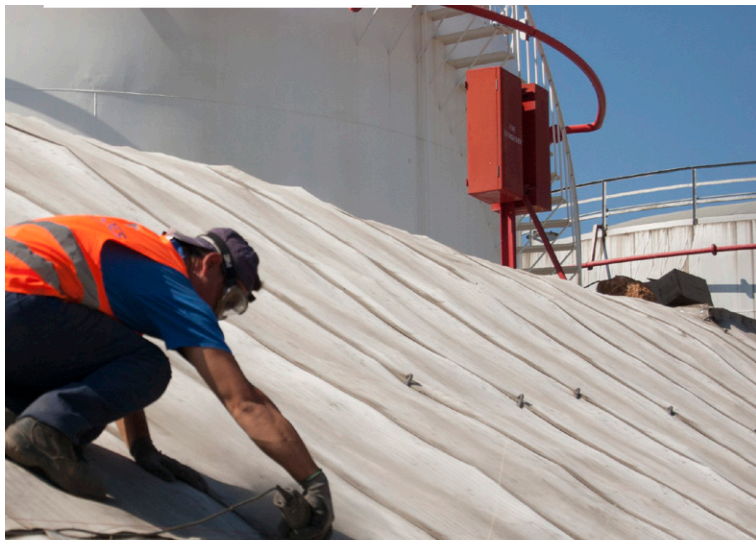
J Pegs (seen right) were also used to fix the CC
