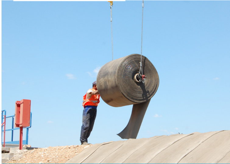
The CC was mounted onto a spreader beam and crane for easy deployment
