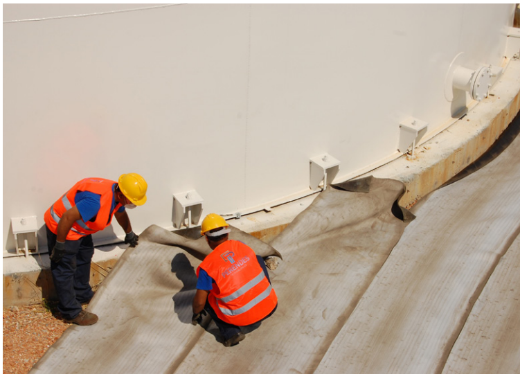
CC was cut using hand tools to negotiate storage tanks
