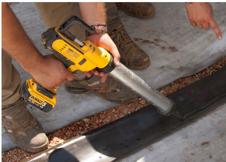
Overlaps of CC were sealed using Everbuild Clearfix adhesive sealant
