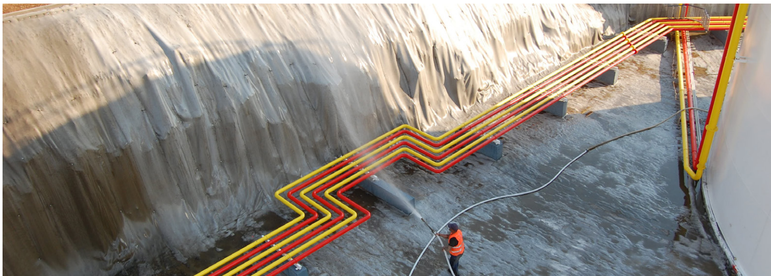
The CC was hydrated using a hose attached to fire pipes
