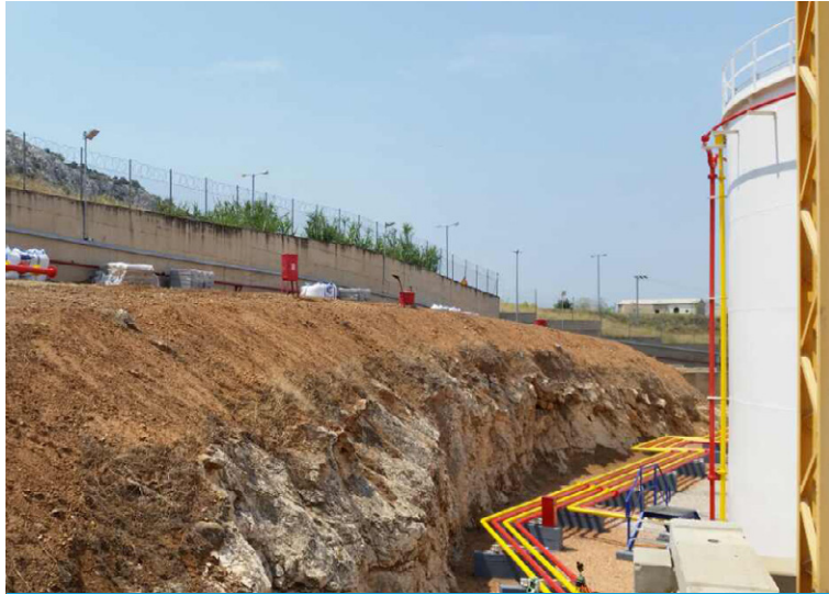
The existing bunds had been affected by weathering erosion
