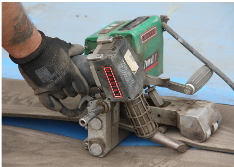
Setting up a thermal welder
