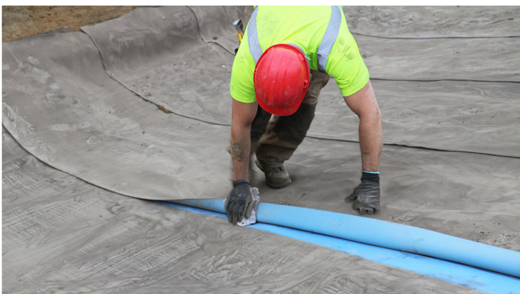
Cleaning the geomembrane faces to be welded
