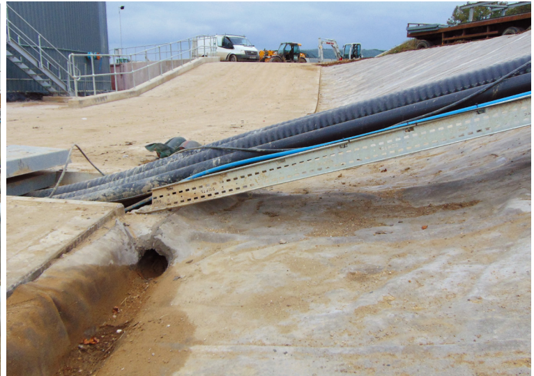
Toe drain details
