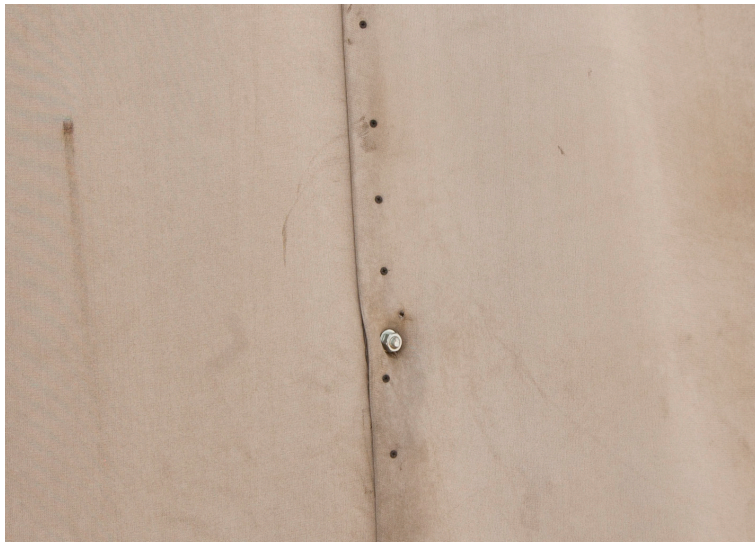
The CC was fixed and jointed using screws and anchor bolts
