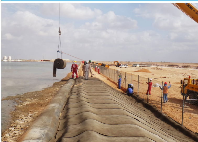
Bulk rolls were mounted on a spreader beam for easy dispensing
