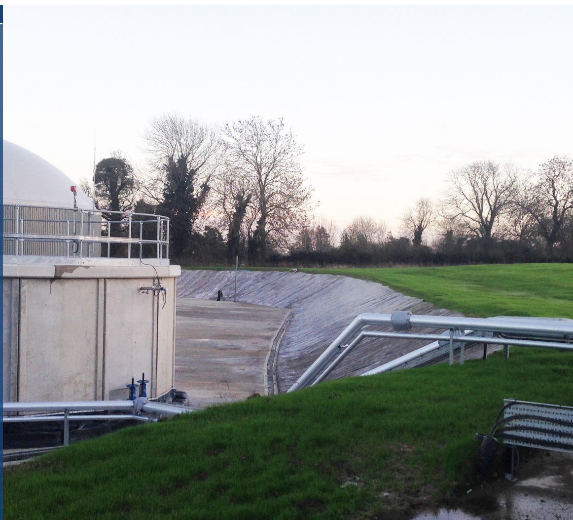
Completed section of bund
