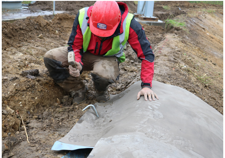
Fixing into the anchor trench
