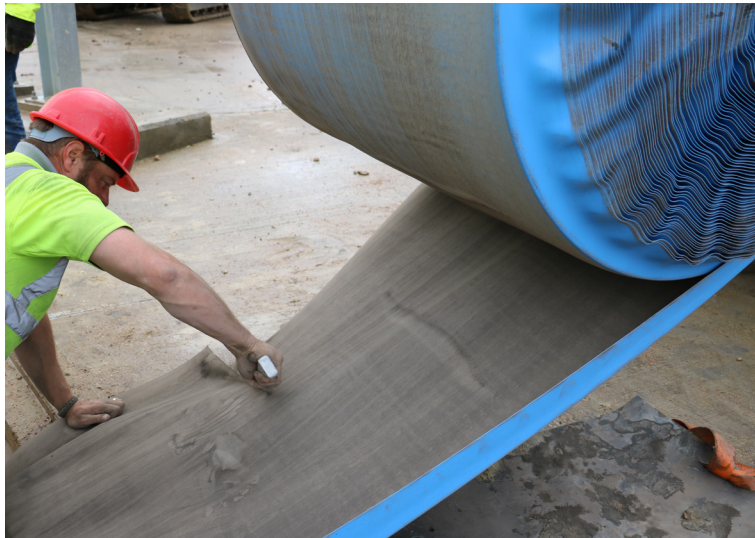
Cutting the CCH to length
