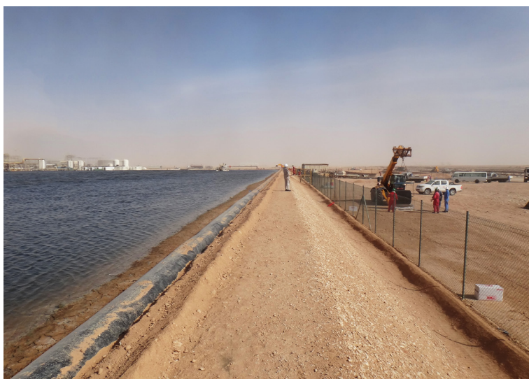
The bund was graded prior to installation
