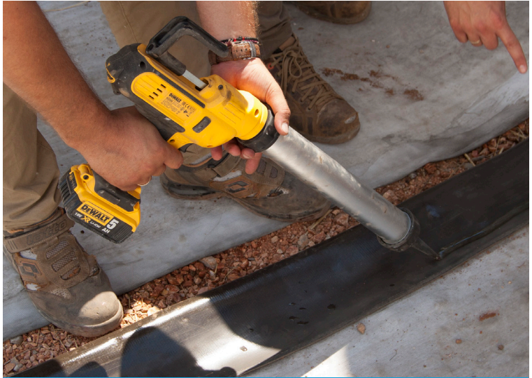
Overlaps were sealed using Everbuild Clearfix adhesive sealant
