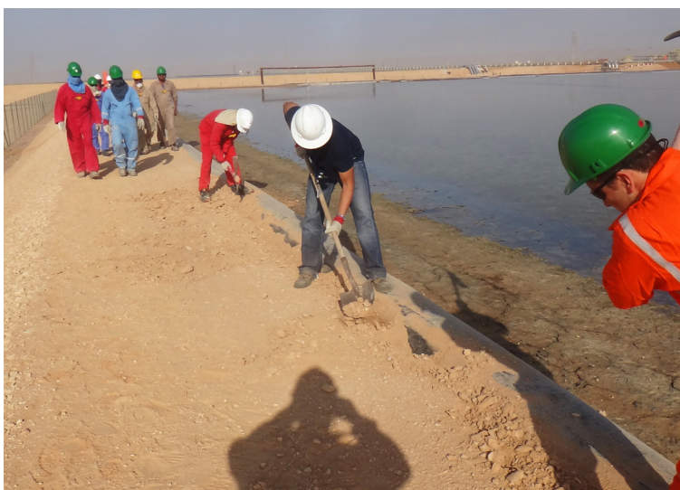
An anchor trench was created prior to installation
