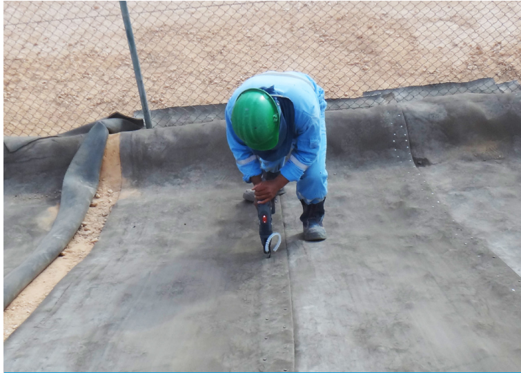
Fixing overlaps with screws
