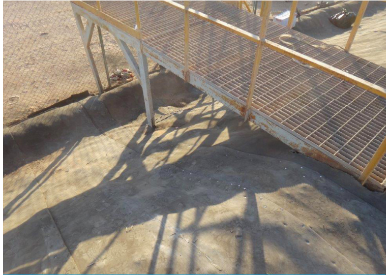
CC installed under a stairway
