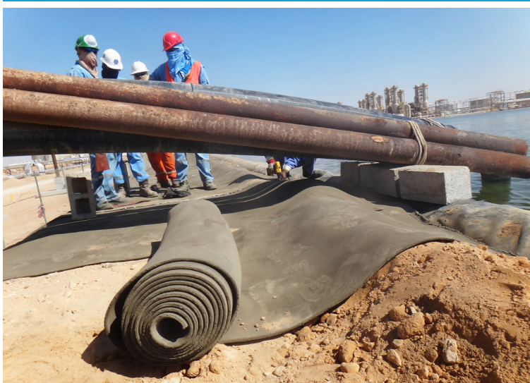
A pre-cut piece of CC being laid under existing pipework
