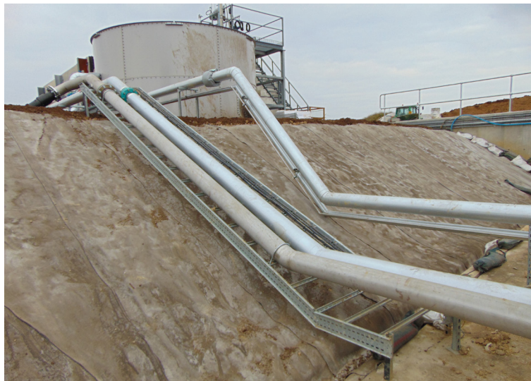
CCH installed around existing infrastructure
