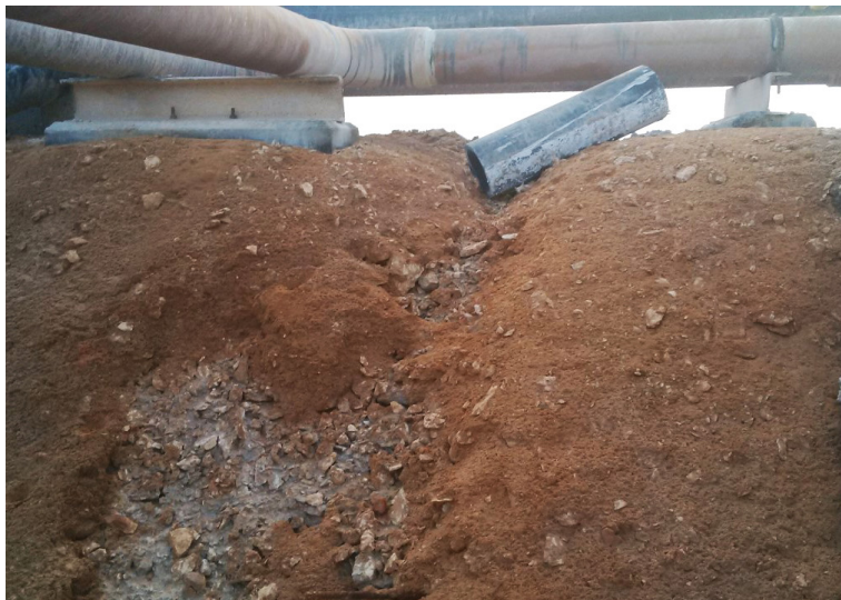
The bund was severely eroded in some areas prior to works
