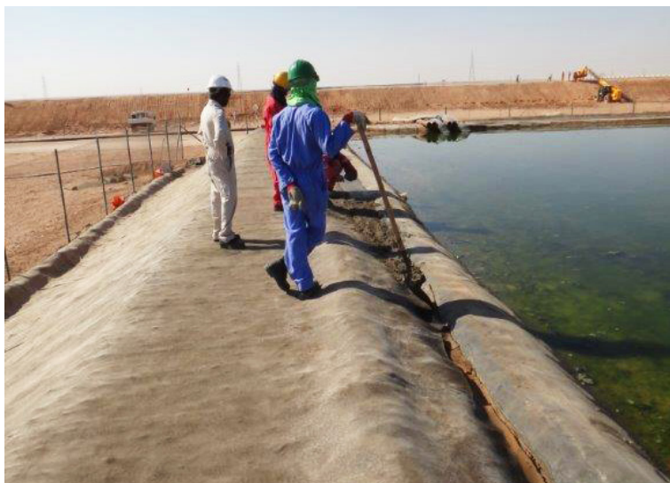
The CC was jointed with screws
