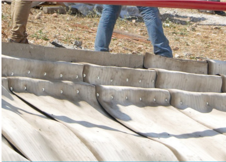
CC was fixed to a concrete slab at the crest of the slope with masonry nails
