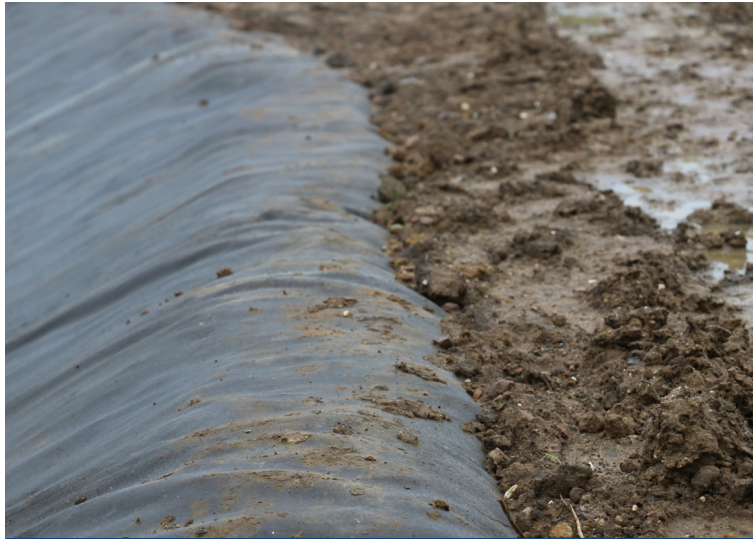
Backfilled anchor trench
