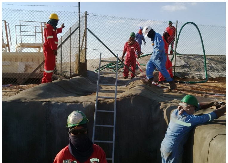
The CC was cut to shape accomodate existing infrastructure
