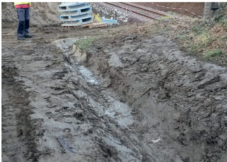
Graded channel prior to installation
