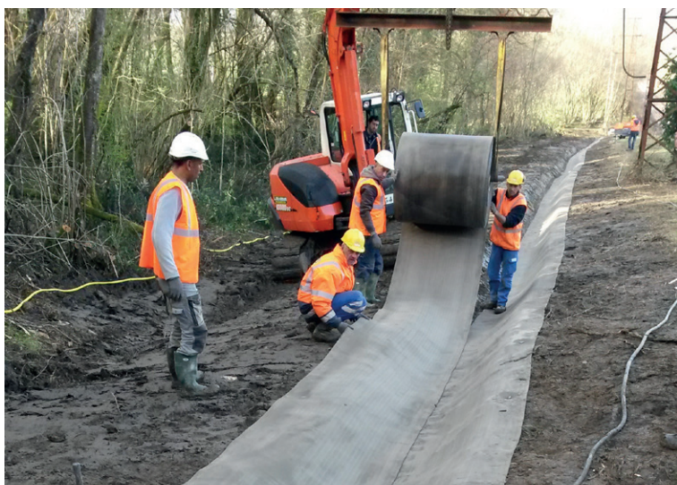
Edge of second layer overlapped the first by 100mm
