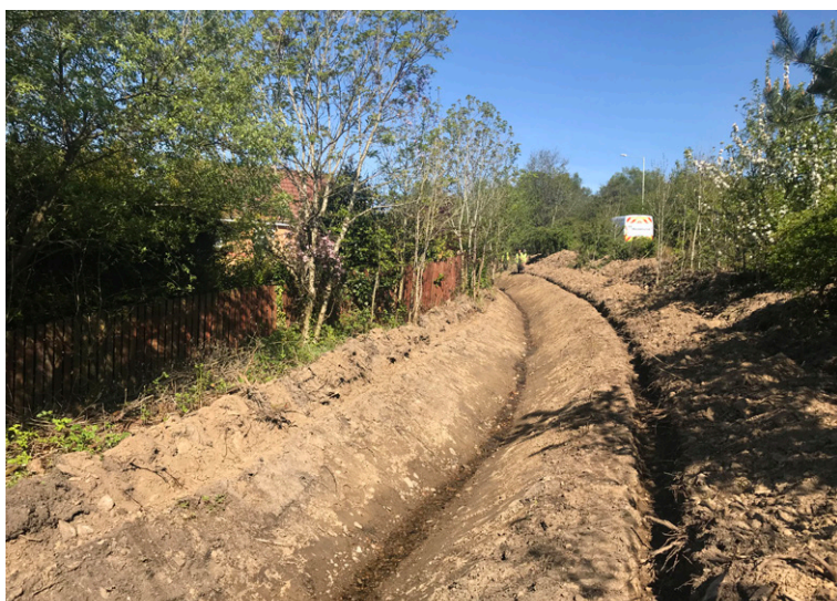
Channel following creation of anchor trenches
