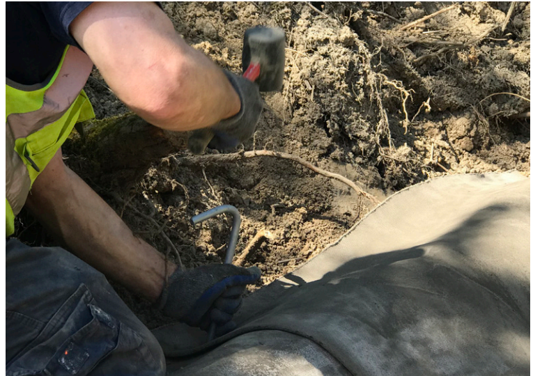
Securing CC edges using ground pegs
