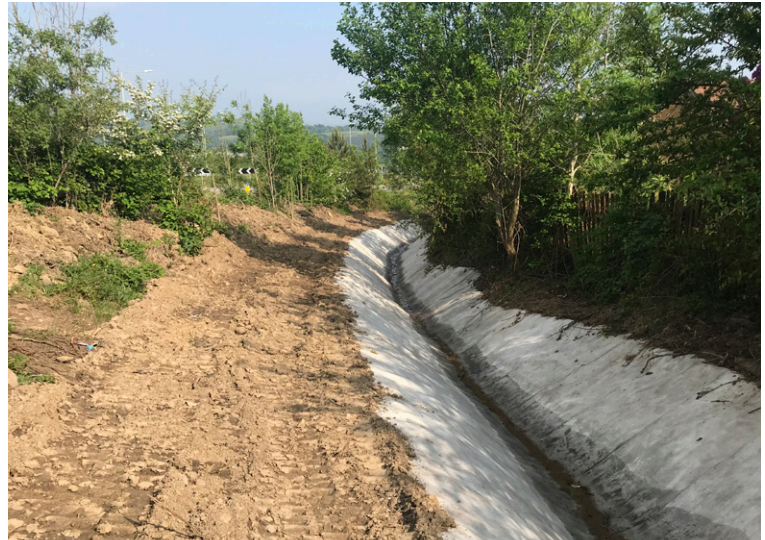
Completed channel following backfilling of anchor trenches
