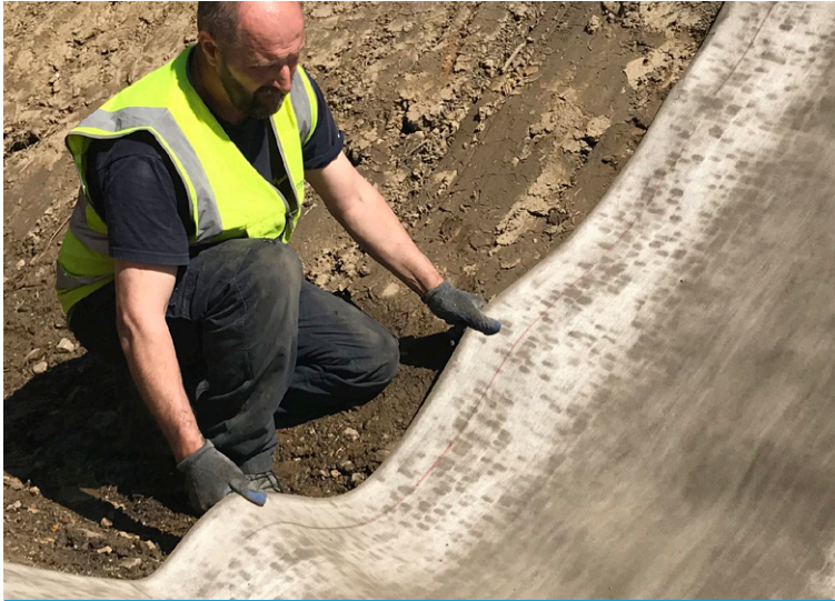
Edges of material marked out for overlap
