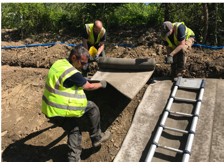
Deployment of CC by hand
