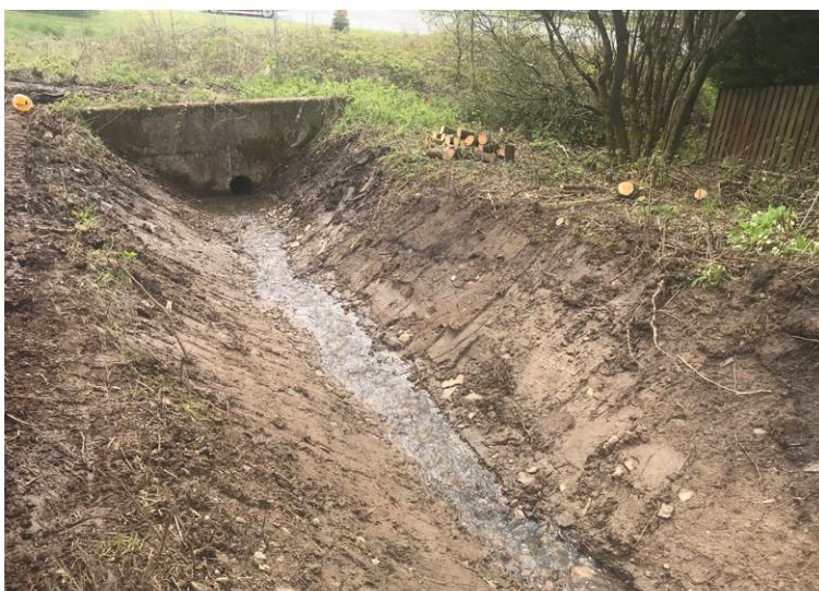
Excavated channel at headwall end
