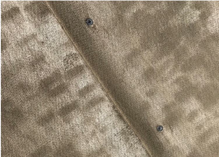
Overlaps jointed using screws
