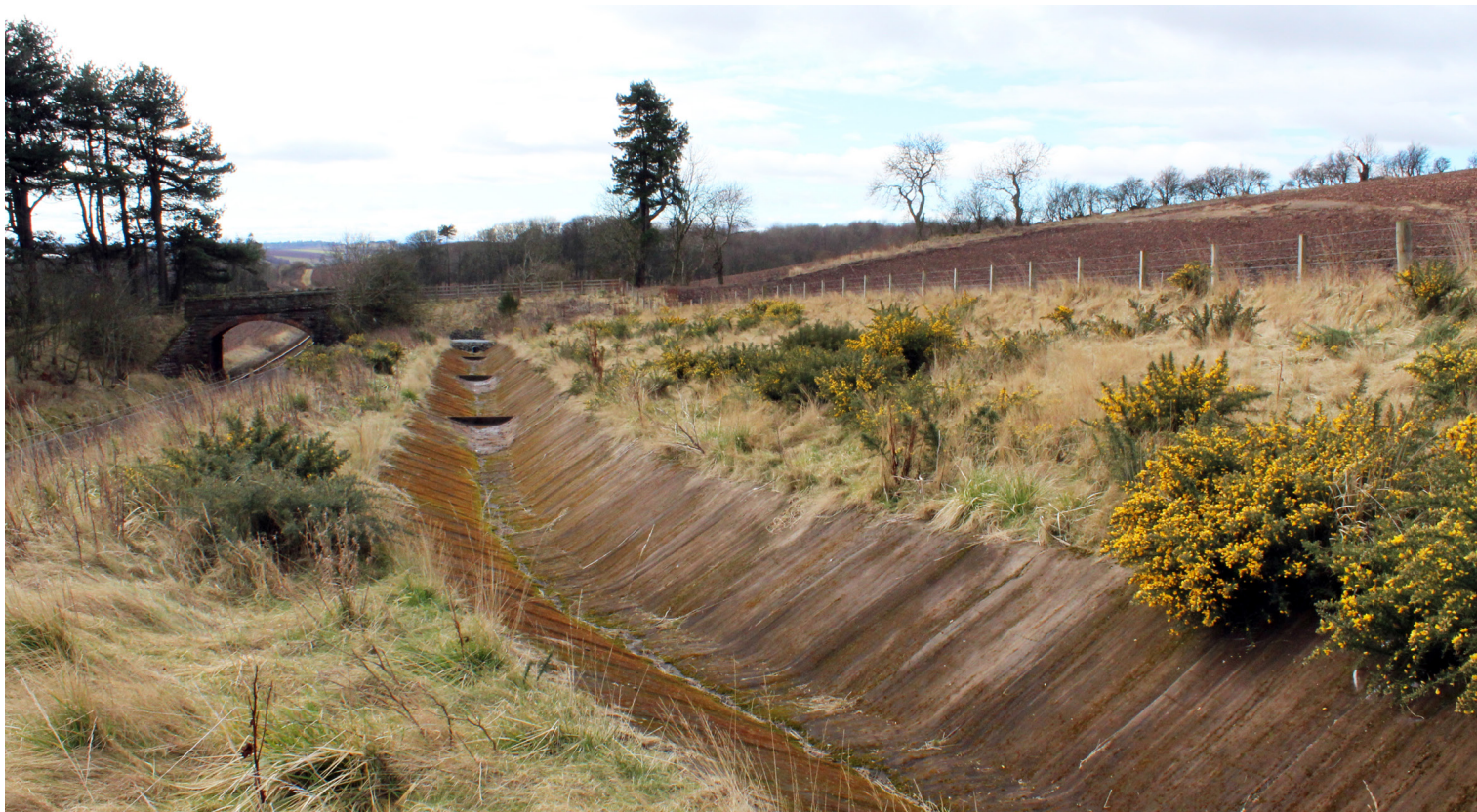
Completed southern section of lined channel, 5 years after installation (2016)
