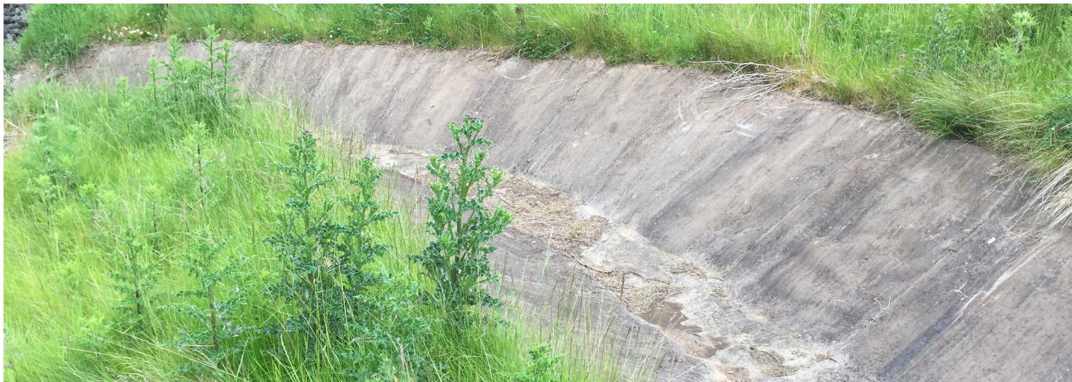
Overspill CC lined ditch section
