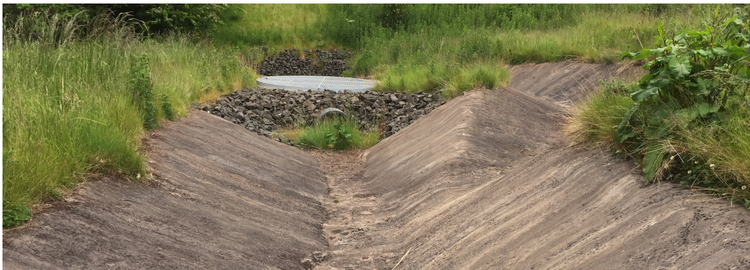
Widest section of ditch, showing overspill route and silt trap entry
