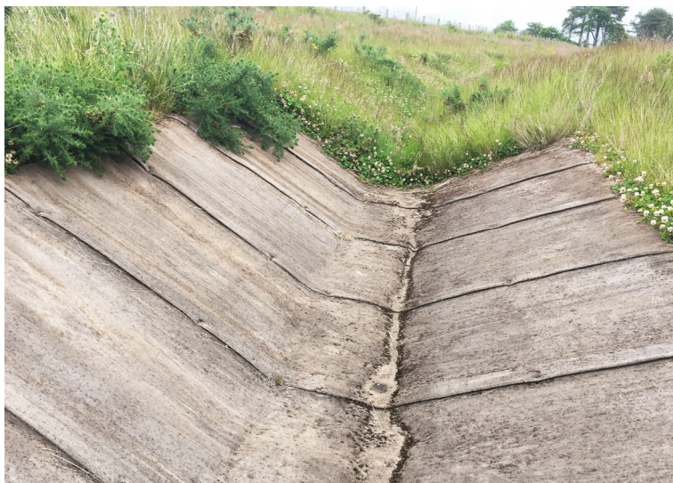
Start of CC lined section, showing vegetation growth on unlined sections
