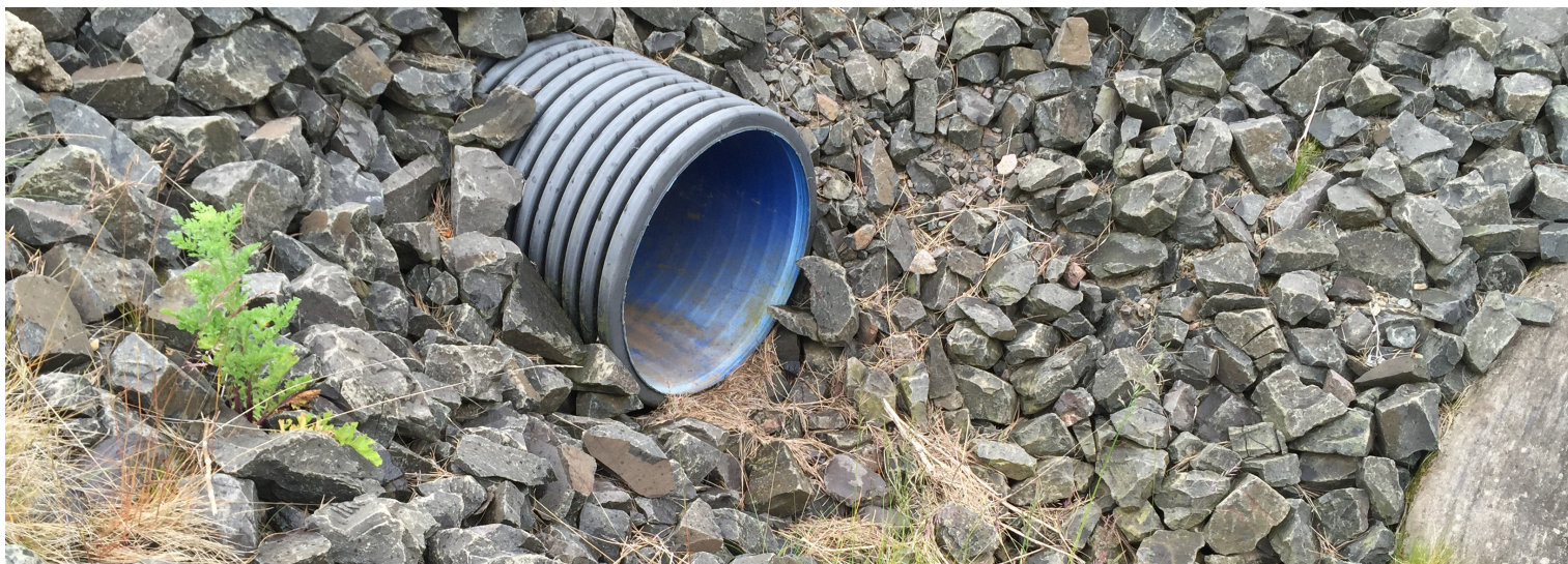
CC lined channel terminating at silt trap outlet
