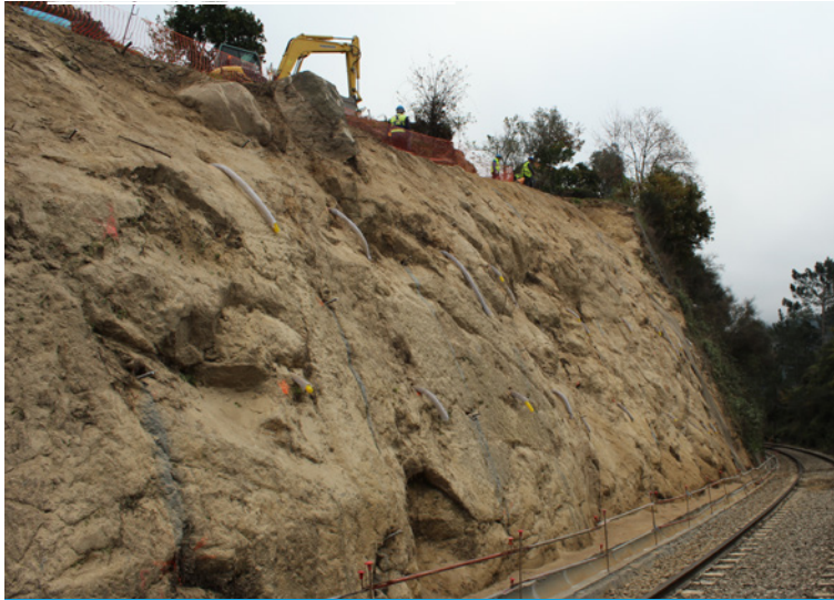
Large rocks, debris and vegetation were removed prior to installation
