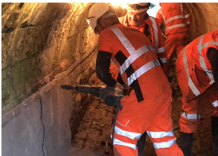
Jointing overlaps using shot-fired nails
