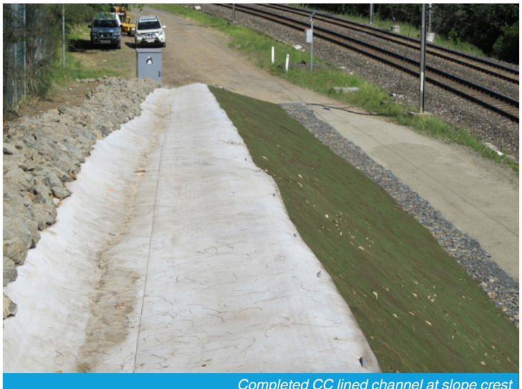
Completed CC lined channel at slope crest
