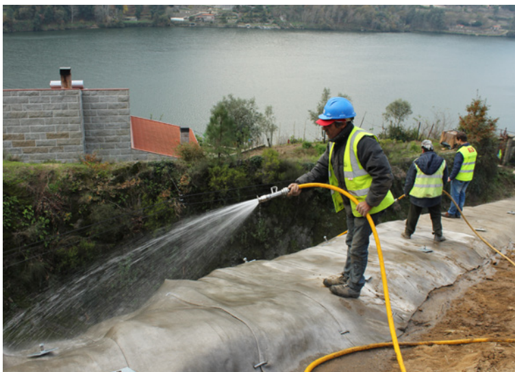
Hydration was given in two stages
