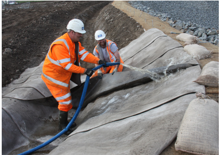
Ground pegs were used to secure the CC in the anchor trenches
