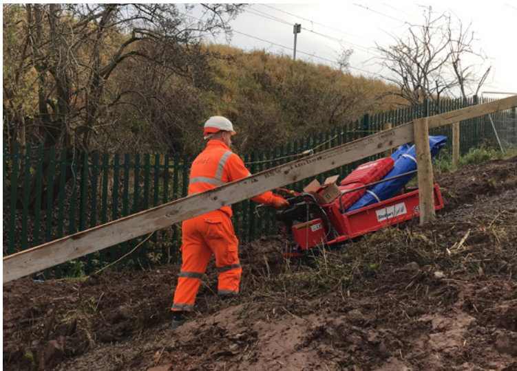
CC batched rolls transported by trolley
