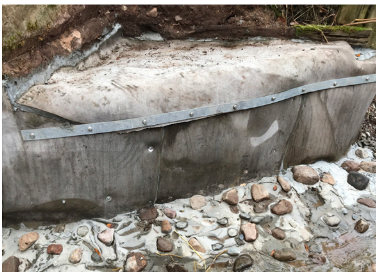
Termination details on wall outside culvert
