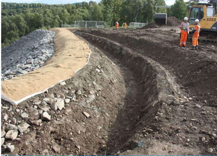
A V bucket was used to dig the channel
