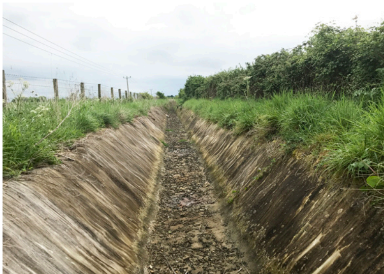
Original CC lined channel installation three years after completion
