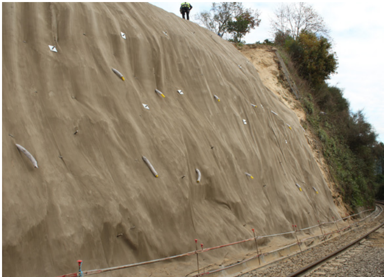
The CC was cut to fit around the pre-fitted weep holes
