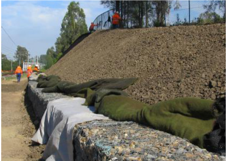
Slope following re-grading and gabion placement
