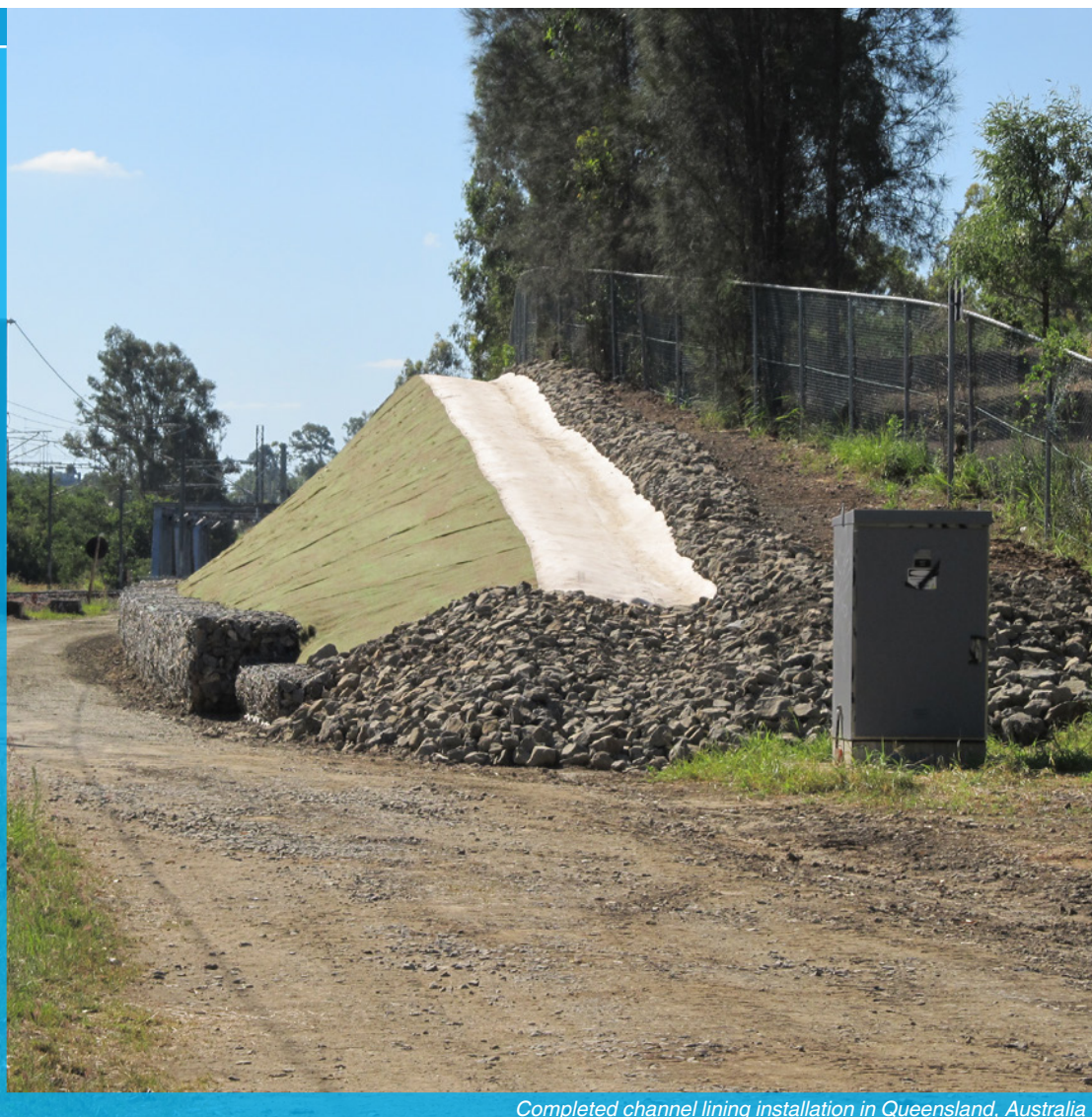
Completed channel lining installation in Queensland, Australia
