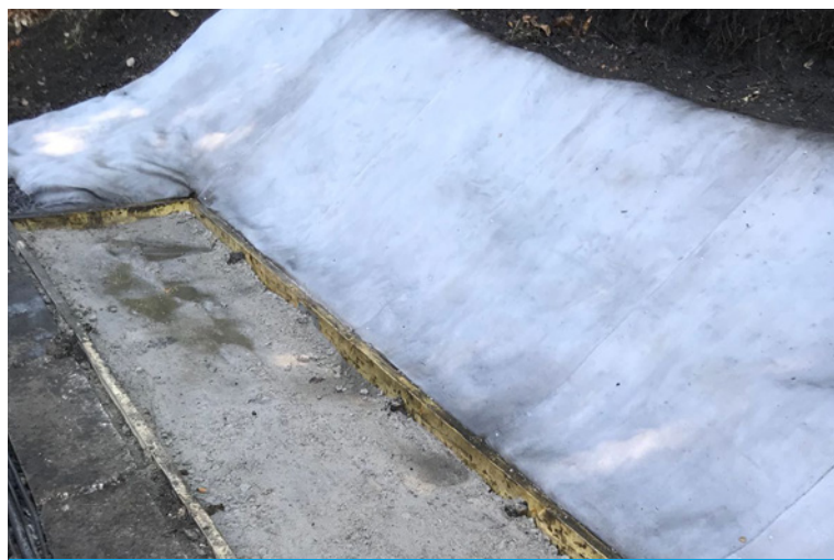
CC installed around framework
