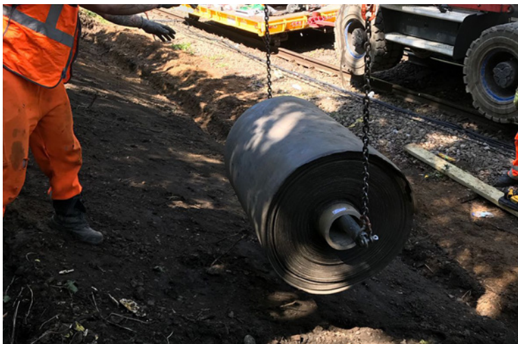
Deploying first length of CC
