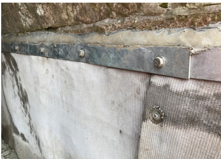
Termination of CC edges using steel bars and grout
