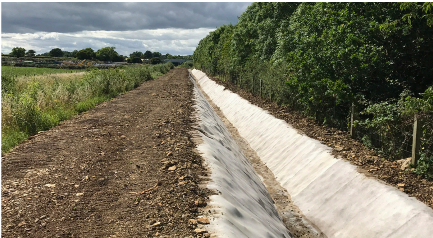
Completed second CC lined channel section in 2017 in Sherston, Wiltshire
