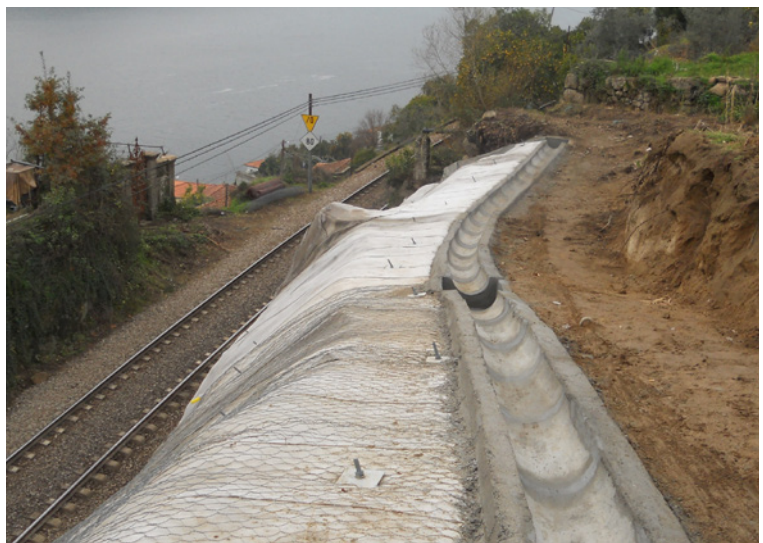
Edges at the crest buried under a poured concrete drainage channel
