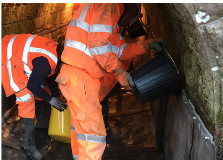
Hydration of CC on culvert walls
