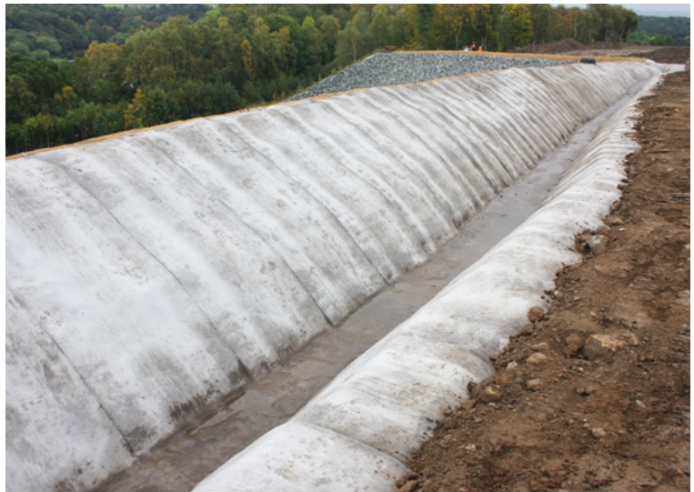
Layers of CC were fixed using stainless steel screws
