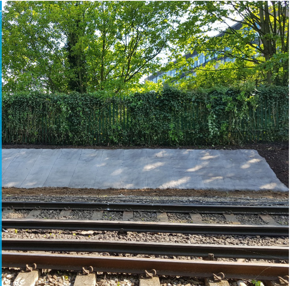
Section of completed CC installation
