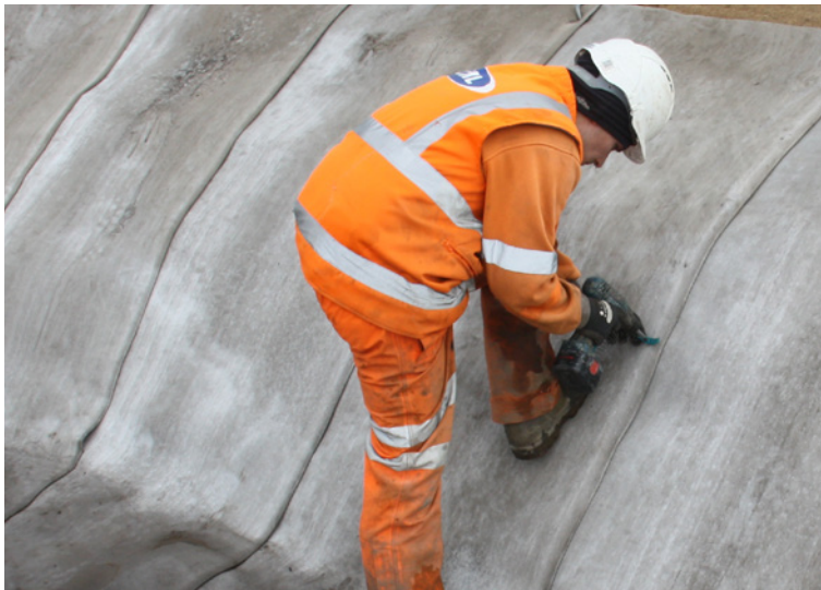
CC under the overlaps were hydrated before fixing
