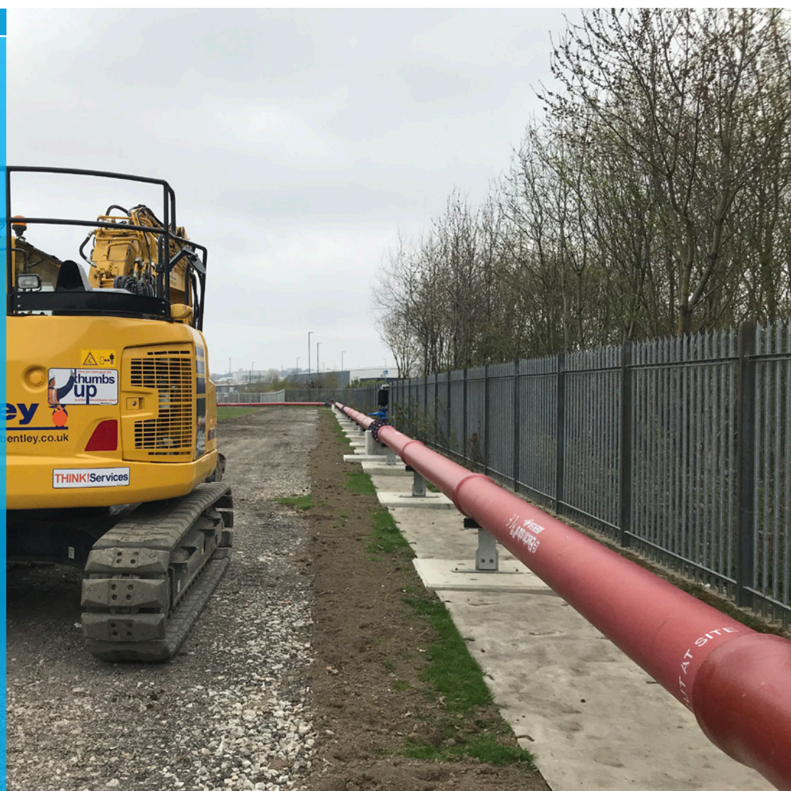
Completed installation of CC5™ around Electrosteel pipeline upstands for weed suppression
