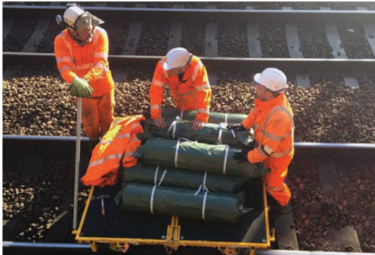
Delivery of CC batched rolls to site area via rail trolley
