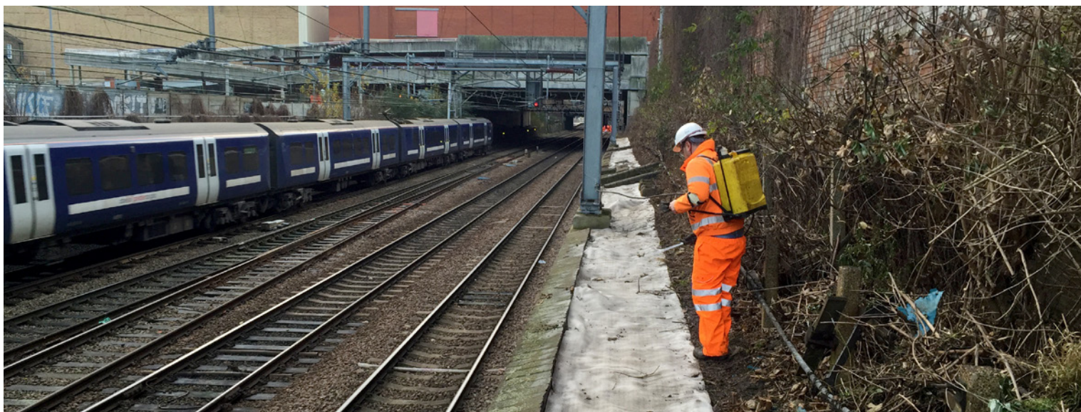
Backfilling anchor trench at toe of second section berm
