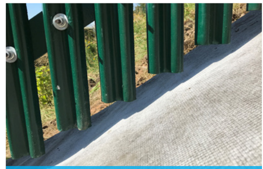
CC installed retrospectively around fencing
