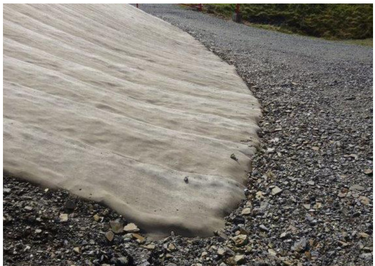
Anchor trenches backfilled following hydration
