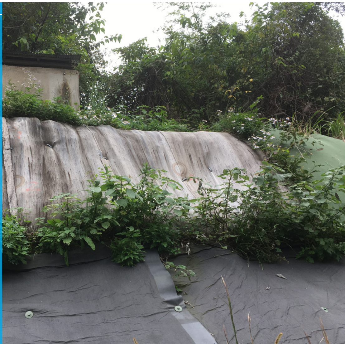
Trial CC section 26 months after installation
