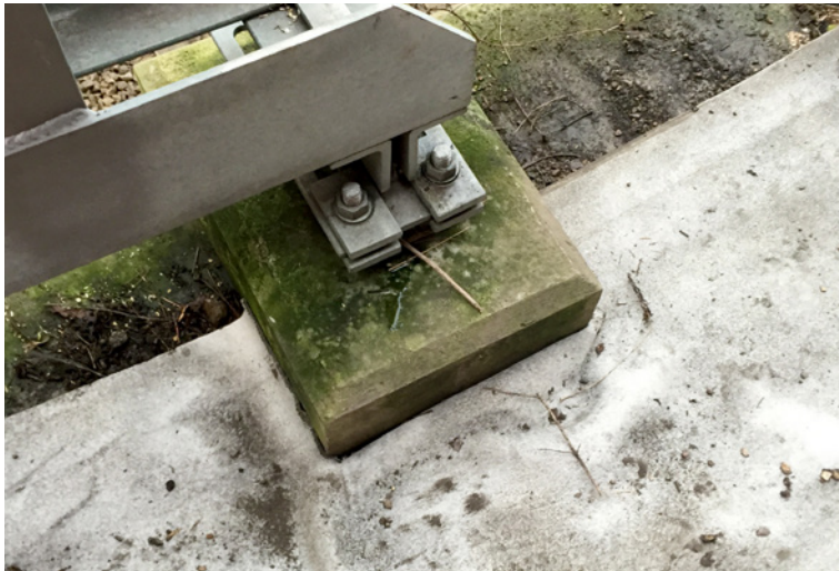
Cutting and detailing of CC to accommodate stanchions and upstands
