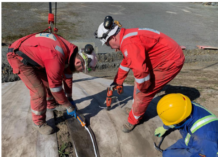
Applying sealant and screwing layers together at 50mm centres
