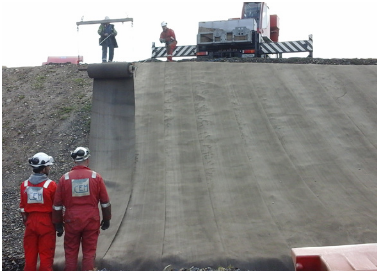
CC secured in toe anchor trench and unrolled up bund height
