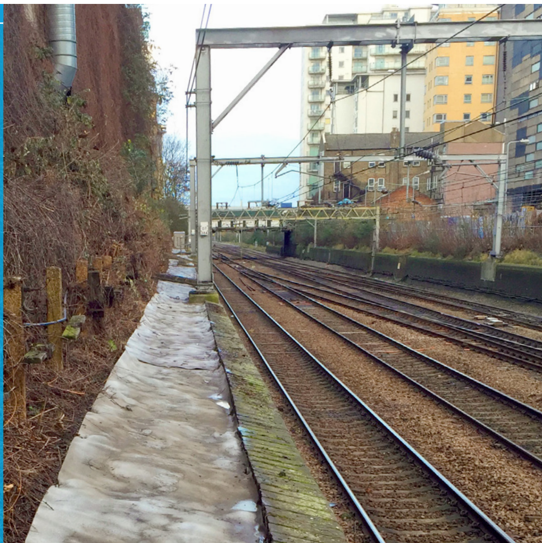
Completed section of lined parapet
