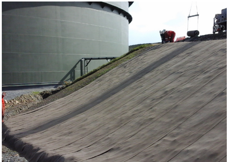
CC layers laid vertically
