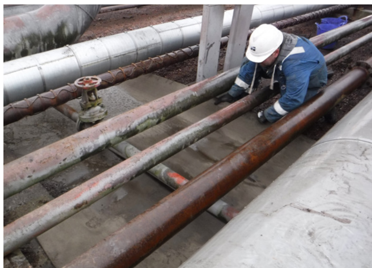
Adjusting position to create 100mm overlaps prior to screwing joint
