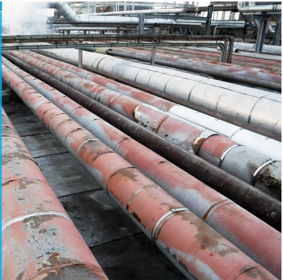
Completed CC lined pipe tracks
