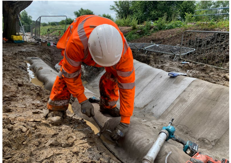
The edge of the CC8™ being pegged at the base of the anchor trench
