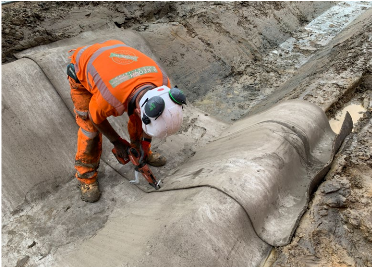
The CC8™ overlapped by 100mm and secured with 30mm screws
