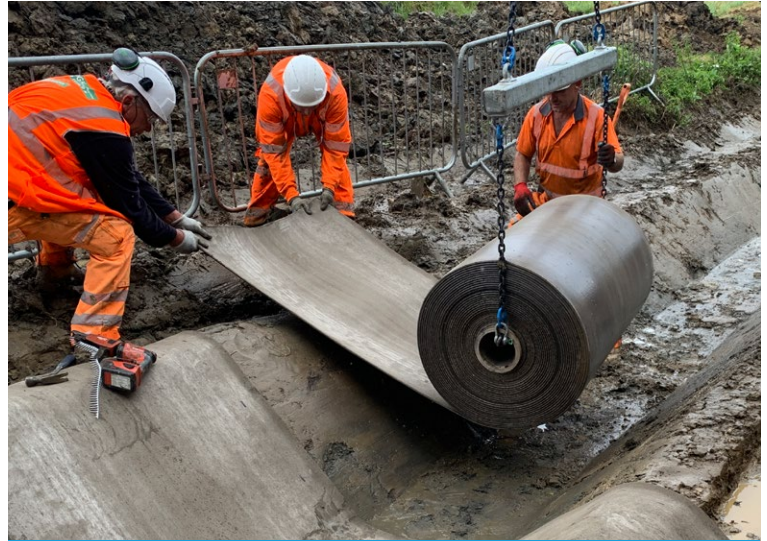
CC8™ suspended from a spreader beam, installed transversely
