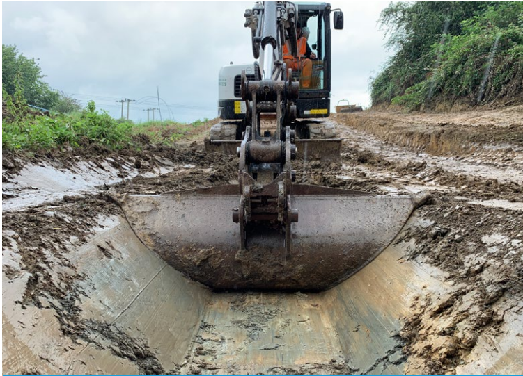
Section of the channel excavated prior to installation
