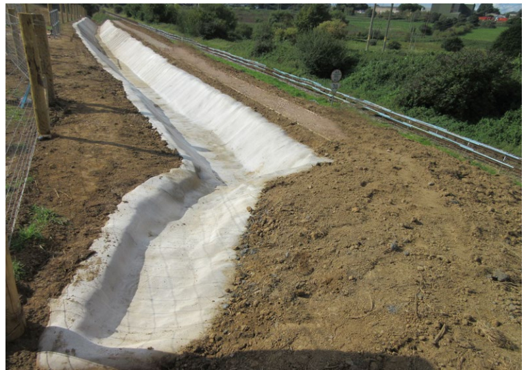
CC8™ installed to accomodate changes in channel profile
