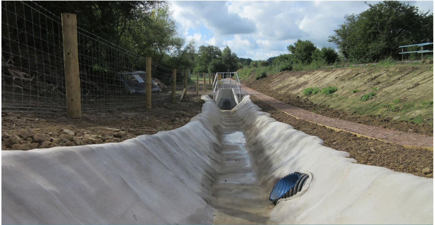
Completed channel lining works
