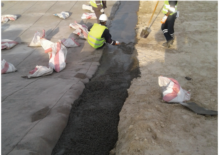
Concrete was poured into the anchor trenches for greater impermeability
