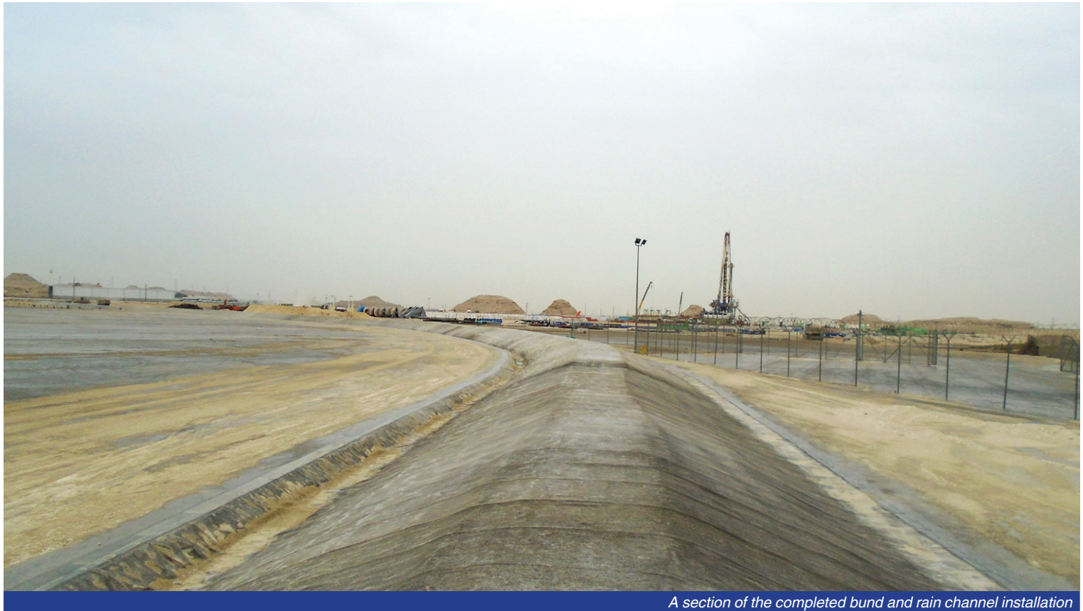
A section of the completed bund and rain channel installation
