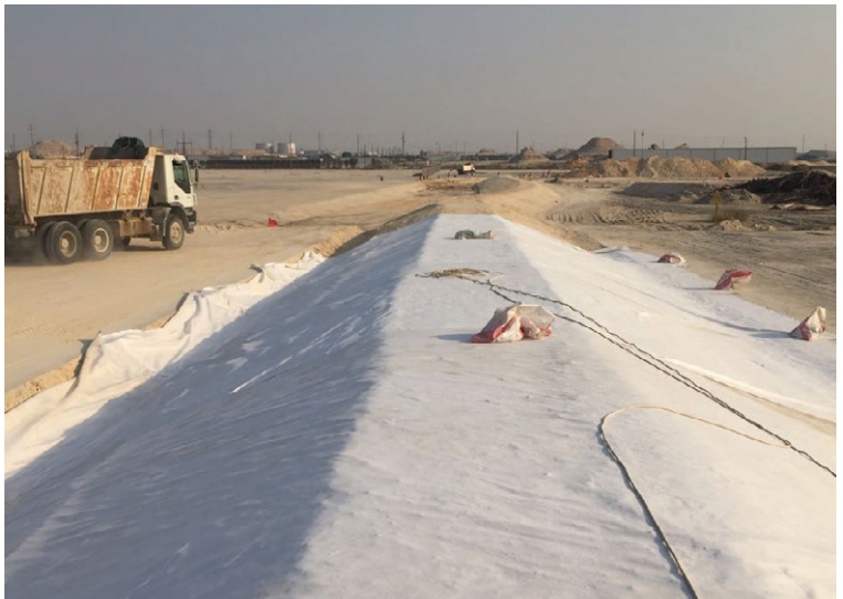
A geotextile was laid over the bund providing a smooth surface for the CCH
