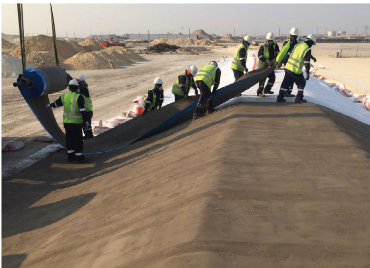
The CCH bulk rolls were mounted onto a spreader beam
