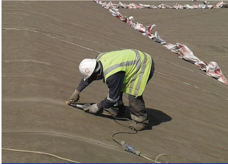
Hot air blower and roller welding method
