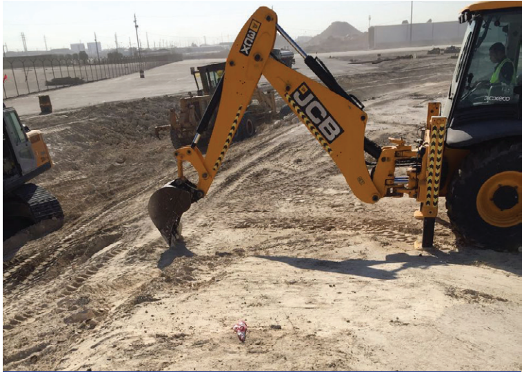
Anchor trenches were dug using a JCB
