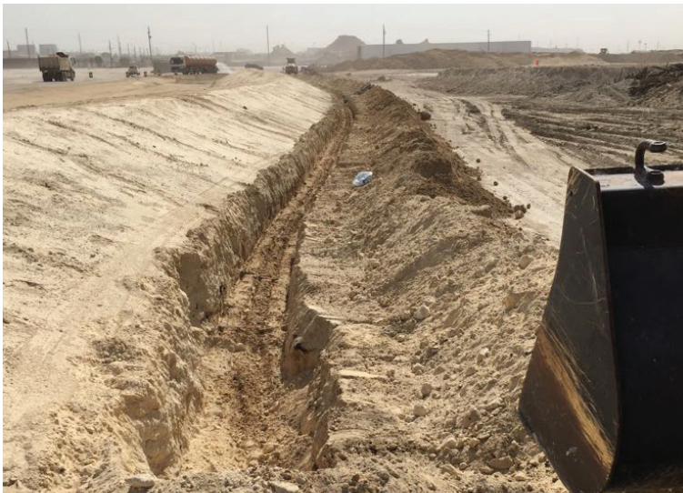
Anchor trenches ready for installation
