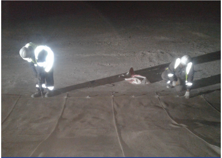
The drilling and bolting of the CCH into the asphalt
