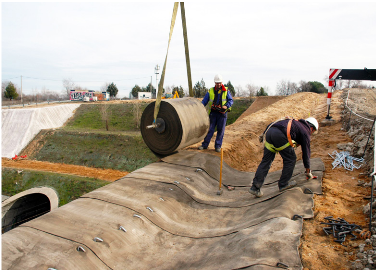
Dispensing from a bulk roll and fixing to top of slope using steel pegs
