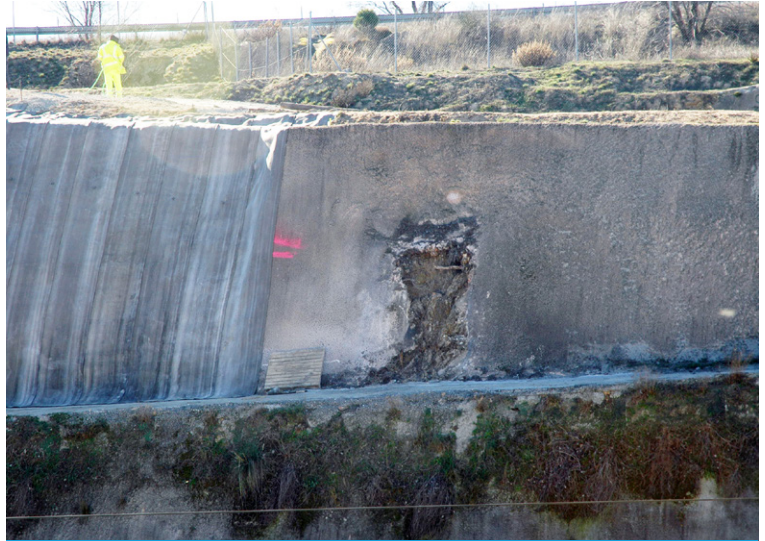
Damaged gunite section from previous remediation work
