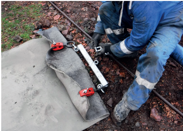
Attachment of low profile pulling jig
