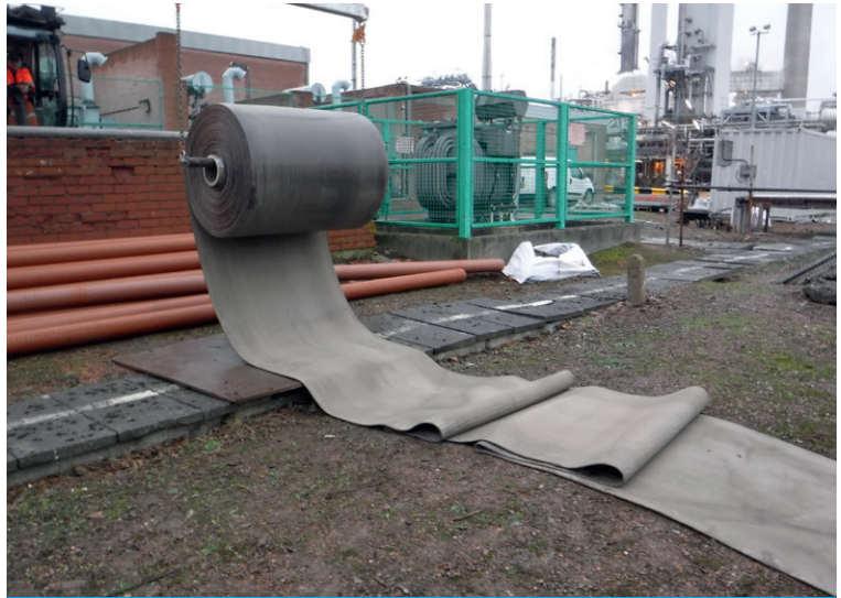
Dispensing of bulk roll CC8 via spreader beam
