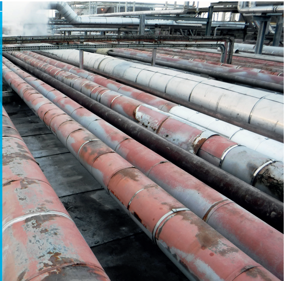
Completed CC lined pipe tracks
