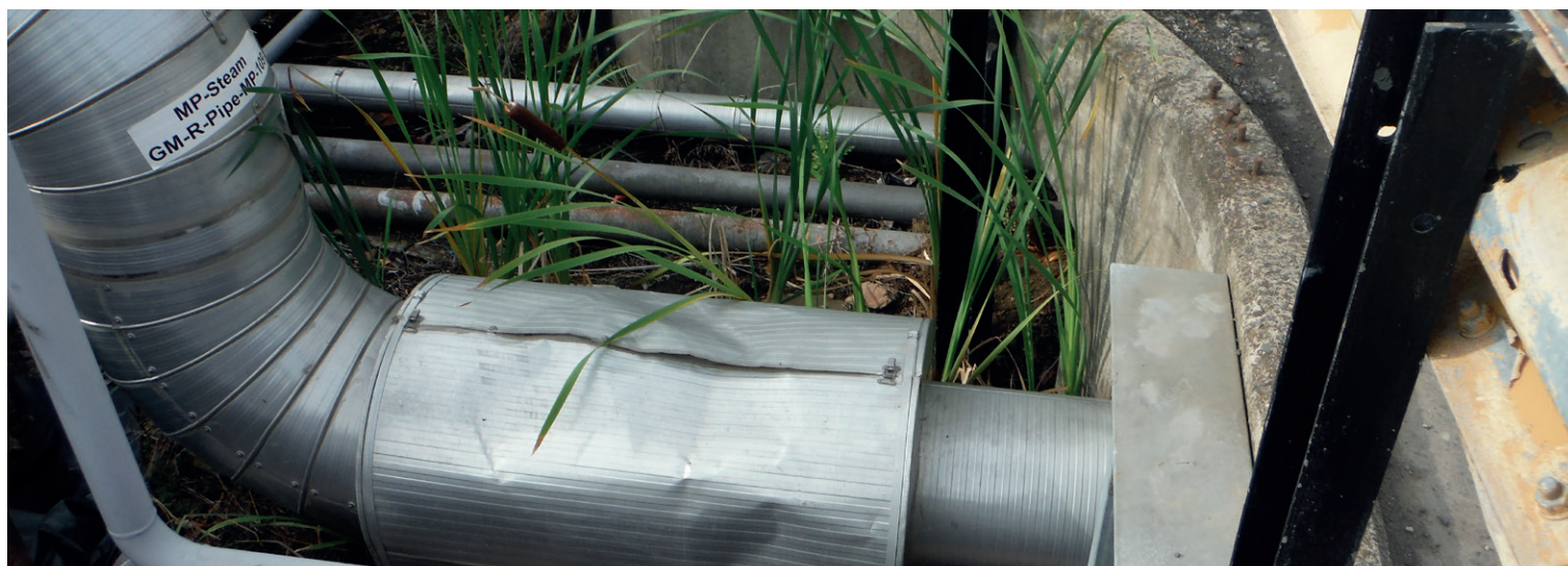
Example of vegetation growth through dilapidated stonechip/ geotextile option
