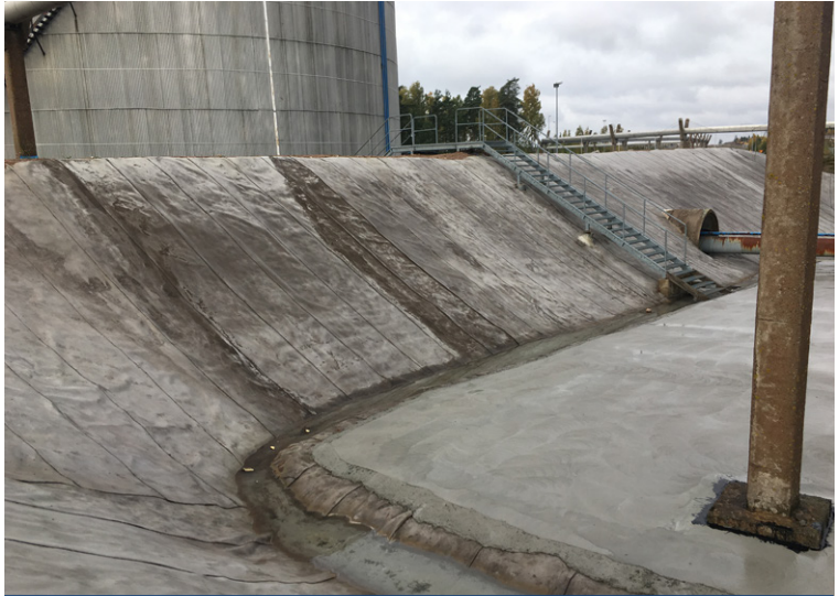
The completed bund installation
