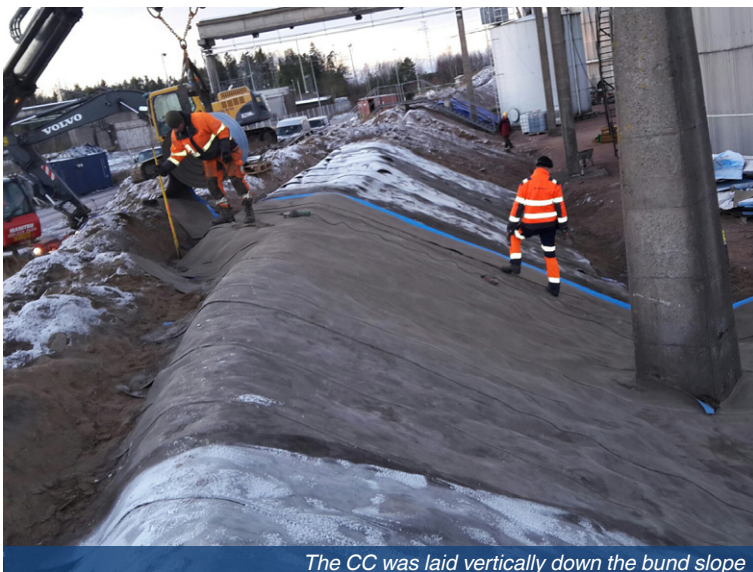
Bund following ground preparation works
