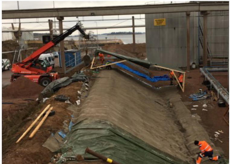
CCH5™ was deployed from an excavator mounted spreader beam
