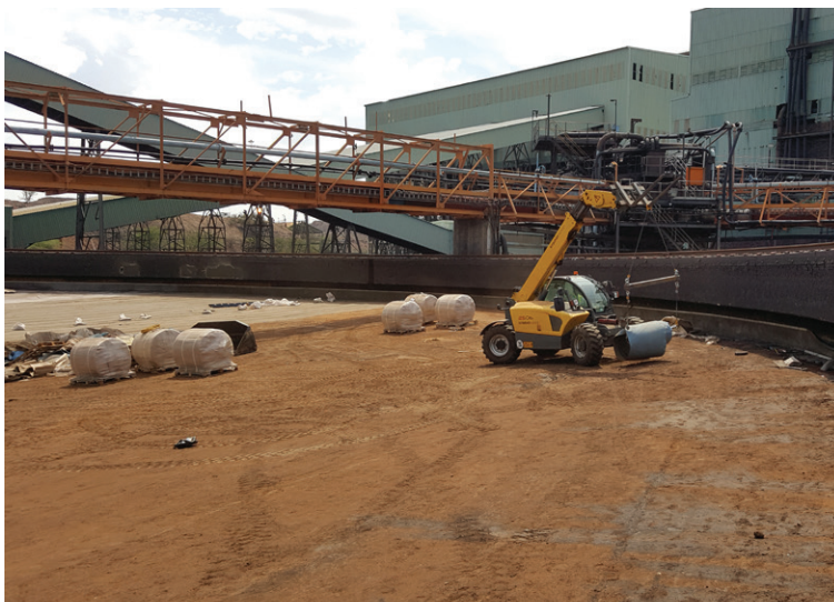
The CCH was delivered to site in bulk rolls
