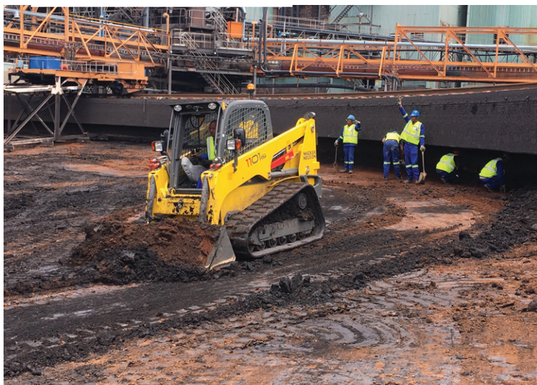
The tank was drawn down and sediment removed before installation
