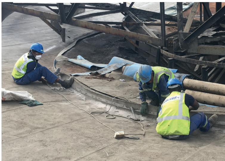
The flexible CC was easily fitted to the complex shape of the tank
