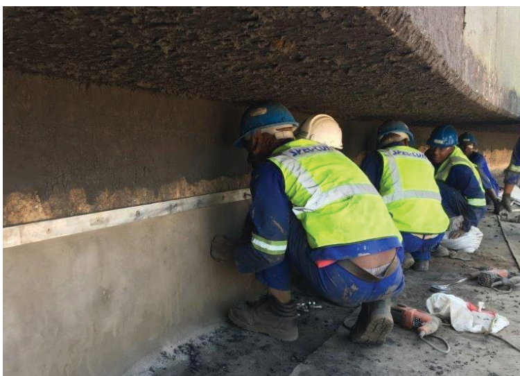
Fixing the CCH to the tank walls
