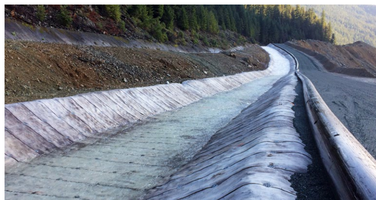
Figure 3. Typical Type II GCCM channel lining application.
