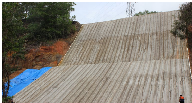
Figure 2. Typical Type I GCCM slope protection application.
