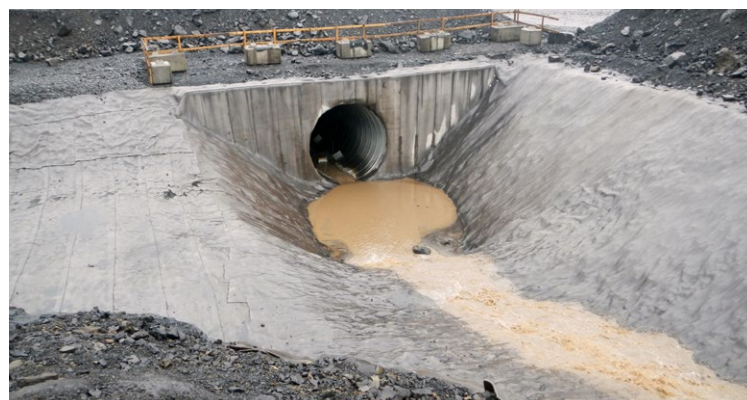
Figure 4. Typical Type III GCCM channel lining application over loose subgrade.
